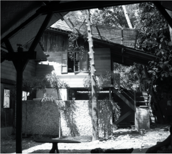
FIGURE 6: Exterior of House Designed by Eko Prawoto
